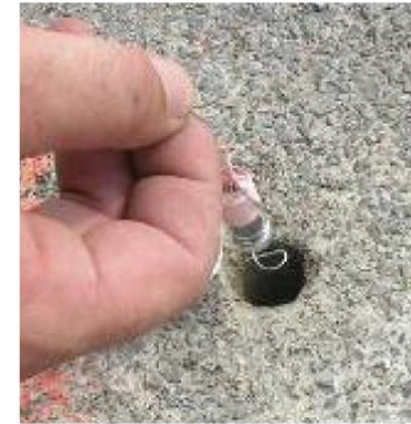
WMS™ Sampler being deployed for sub-slab gas sampling
