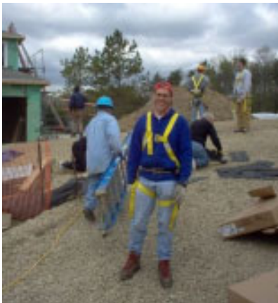
Mark Chapin prepares for roof duty.
