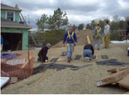
Hey Mark, the ladder to the roof is the other way.
