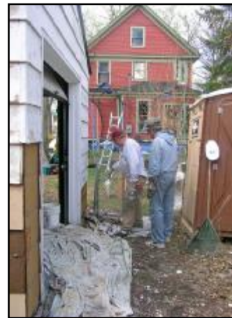
Replacing rotted siding
