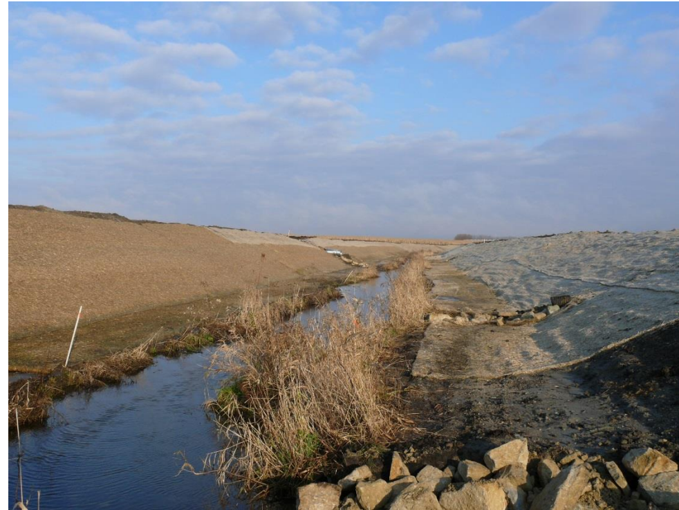
Two-stage drainage ditch
